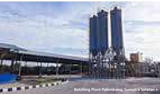
Batching Plant Palembang, Sumatra Selatan •
