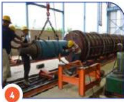
4 Penarikan Besi Prategang Prestressing Iron Withdrawal
