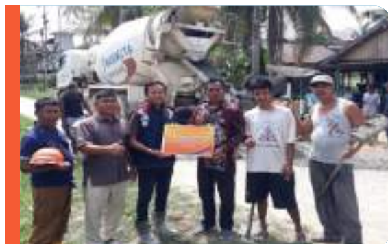
25 Oktober 2023 | October 25, 2023 Perbaikan Jalan di Sepaku Road Repair in Sepaku
