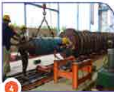
4 Penarikan Besi Prategang Stressing Iron Withdrawal
