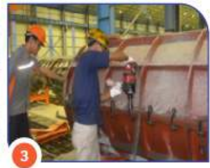
3 Pengecoran Beton & Penutupan Cetakan Concrete Casting & Mold Closure
