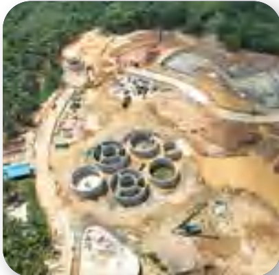
Pembangunan Instalasi Pengolahan Air Limbah (IPAL) KIPP IKN, Kalimantan Timur Construction of Wastewater Treatment Plant (IPAL) KIPP IKN, East Kalimantan
