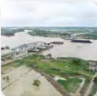
Jembatan Musi Sumatra Selatan Musi Bridge South Sumatra
