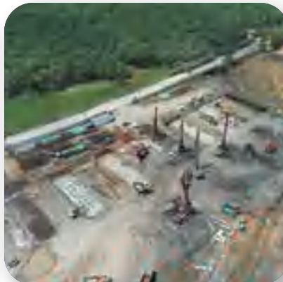
Pembangunan Jalan Akses Bandara VVIP IKN, Kalimantan Timur Construction of VVIP Airport Access Road - IKN, East Kalimantan
